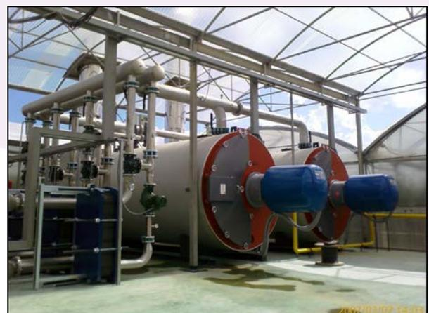
Boiler room (GLP) with exchangers for PVC heating.
